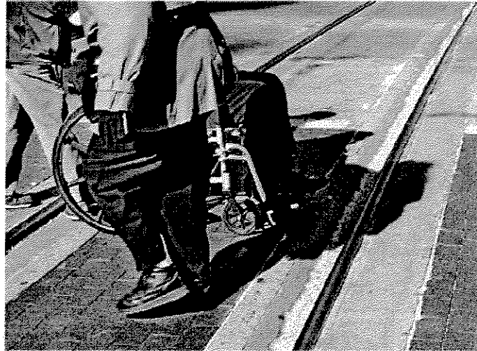
Figure 17 - Flangeway with excessive width that is incompatible with small wheels in a pedestrian crossing area.
