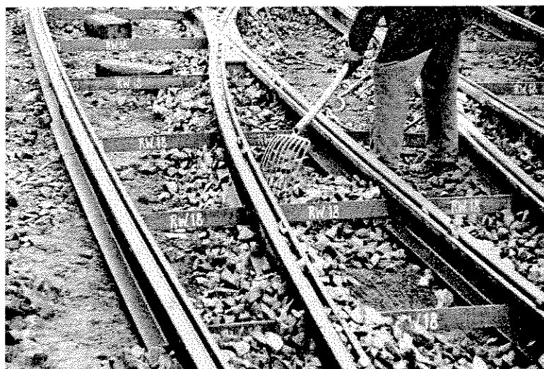
Figure 16. - Typical gauge bar application in a turnout.
