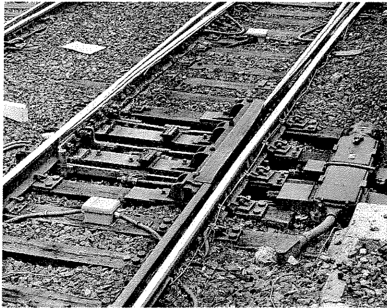
Figure 19. - Turnout with housed point.
